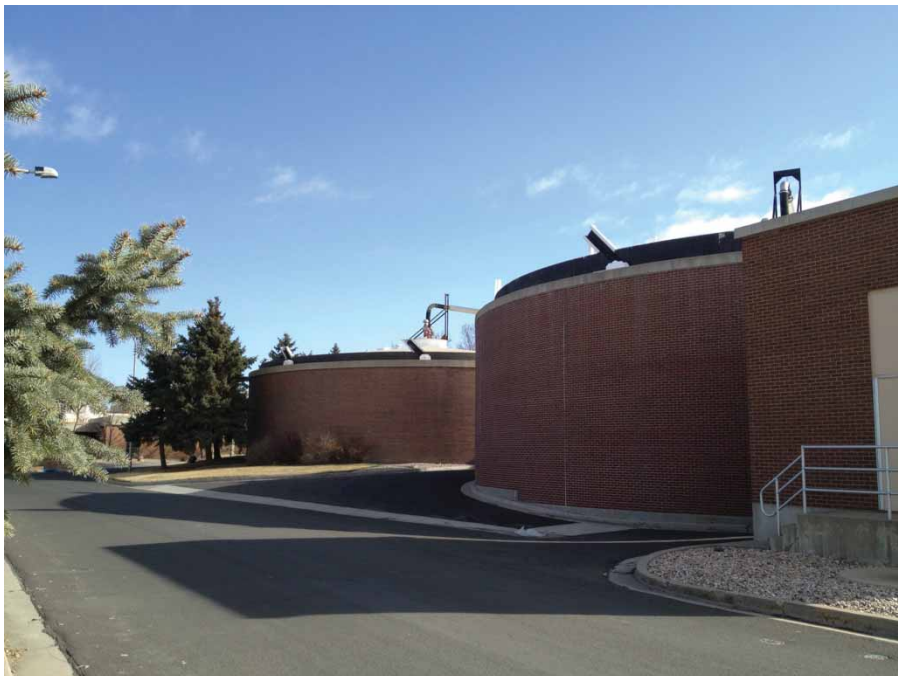
Figure 3 | Fort Collins, Colorado WWTP anaerobic digesters.
