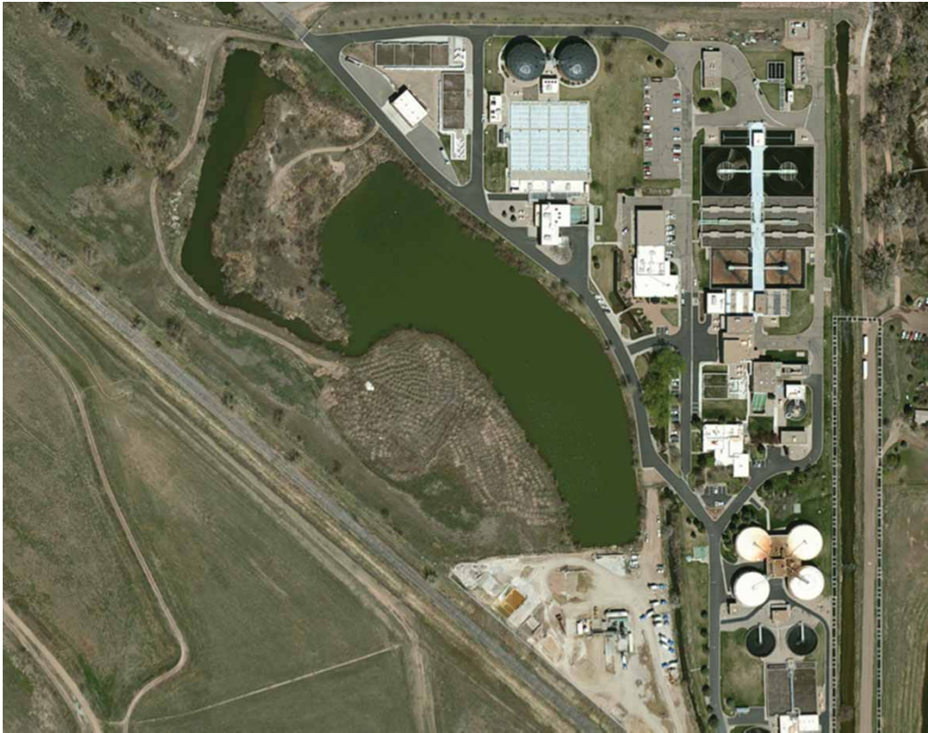
Figure 2 | Aerial view of fort Collins, Colorado WWTP.
